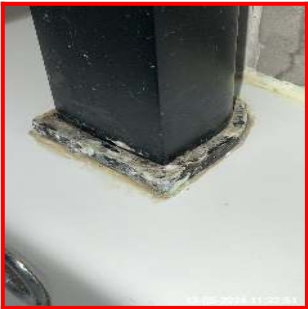
11.4.1 Limescale To Tap Spout And Base
