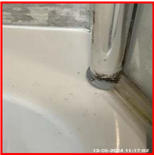
9.5.2 Limescale To Wall Bracket
