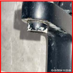
11.4.1 Limescale To Tap Spout And Base
