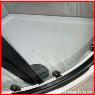
11.5.1 Lift Water Staining To Glass Screen
