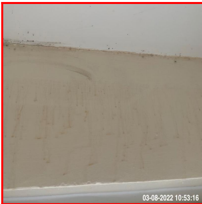
5.4.3 Water Staining / Drip Stains Above Door
