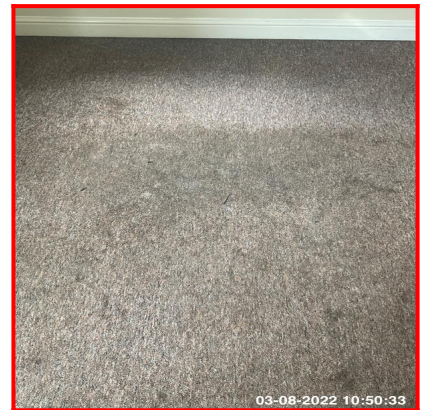
4.9.1 Excess Wear And Staining To Middle Area
