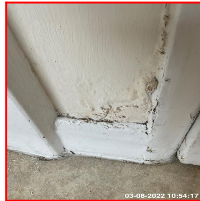
5.4.3 Paint Blistering To Lower Area By Door
