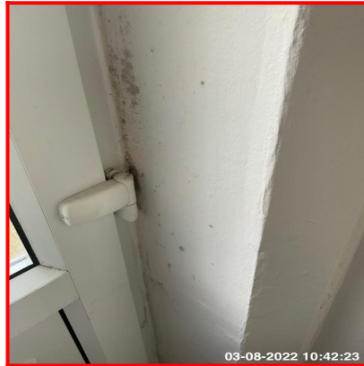
3.3.2 Mildew To Door Reveal Sides And Upper Area
