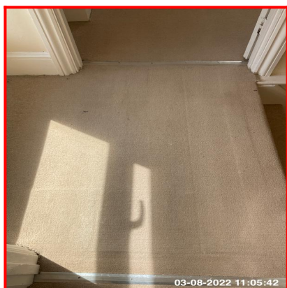
8.7.1 Heavy Wear To Traffic Area At Top
