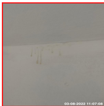
9.4.3 Water Staining Marks To RHS Wall 9.4.3 Water Staining Marks To RHS Wall
