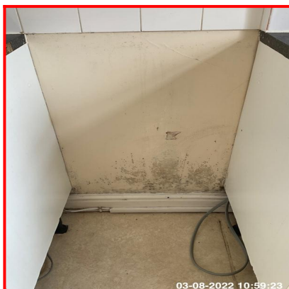
7.4.3 Heavy Mildew Spotting Top RHS And Front Wall
