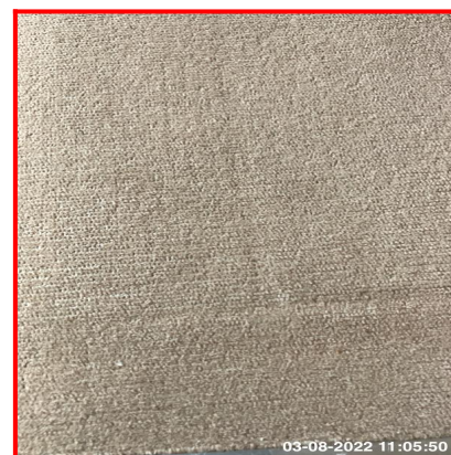
8.7.1 Heavy Wear To Traffic Area At Top
