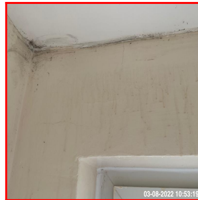
5.4.3 Water Staining / Drip Stains Above Door
