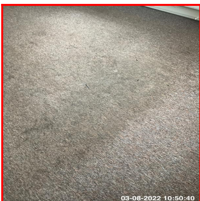
4.9.1 Excess Wear And Staining To Middle Area
