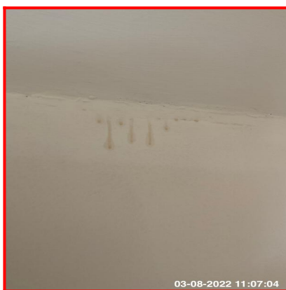
9.4.3 Water Staining Marks To RHS Wall 9.4.3 Water Staining Marks To RHS Wall
