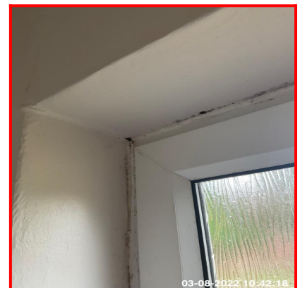
3.3.2 Mildew To Door Reveal Sides And Upper Area
