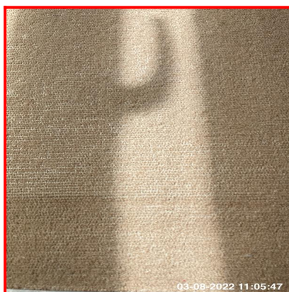
8.7.1 Heavy Wear To Traffic Area At Top
