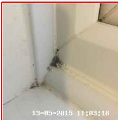
3.5.2 Mould Stains To Seal In Corners
