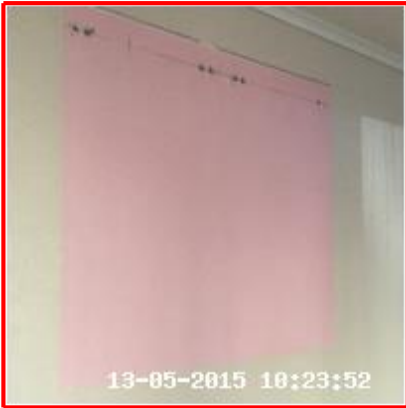
2.4.2 3x Unpainted Patches With Raw Plugs
