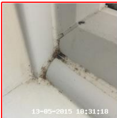
2.5.2 Mould Stains To Seal In Corners
