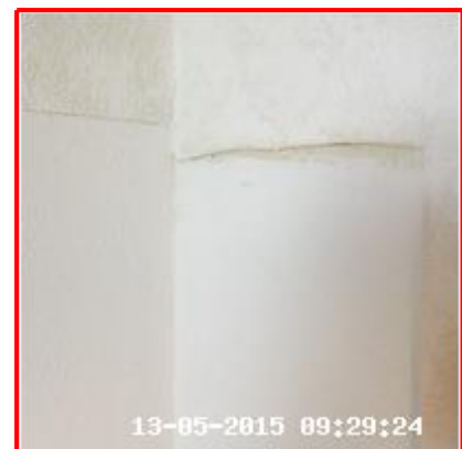
1.4.2 Paper Missing And Paper Peeling Mid Height RHS Of Front Door
