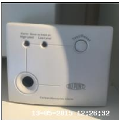
4.16 Carbon Monoxide Detector
