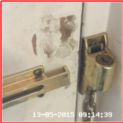
1.1.1 Paint Worn Under Yale Lock
