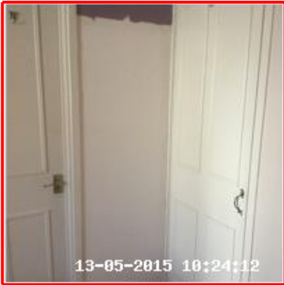
2.4.2 3x Unpainted Patches With Raw Plugs
