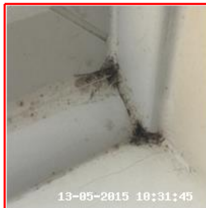
2.5.2 Mould Stains To Seal In Corners
