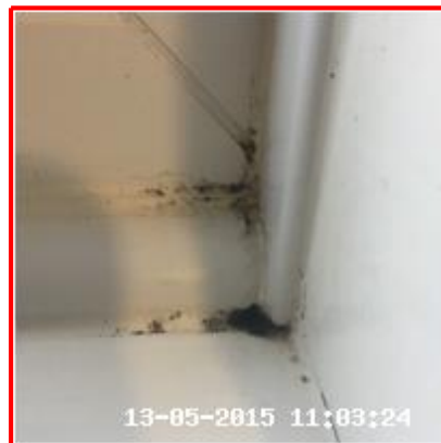
3.5.2 Mould Stains To Seal In Corners
