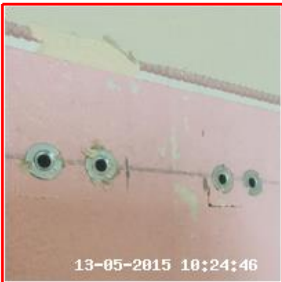
2.4.2 3x Unpainted Patches With Raw Plugs
